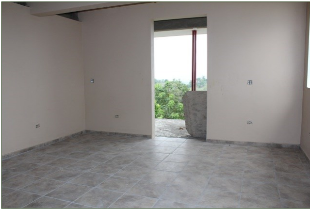
Paint on the walls and ceramic on the floor of the residence living room
